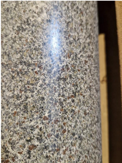
Figure 5. Renaissance wax sheen detail.
