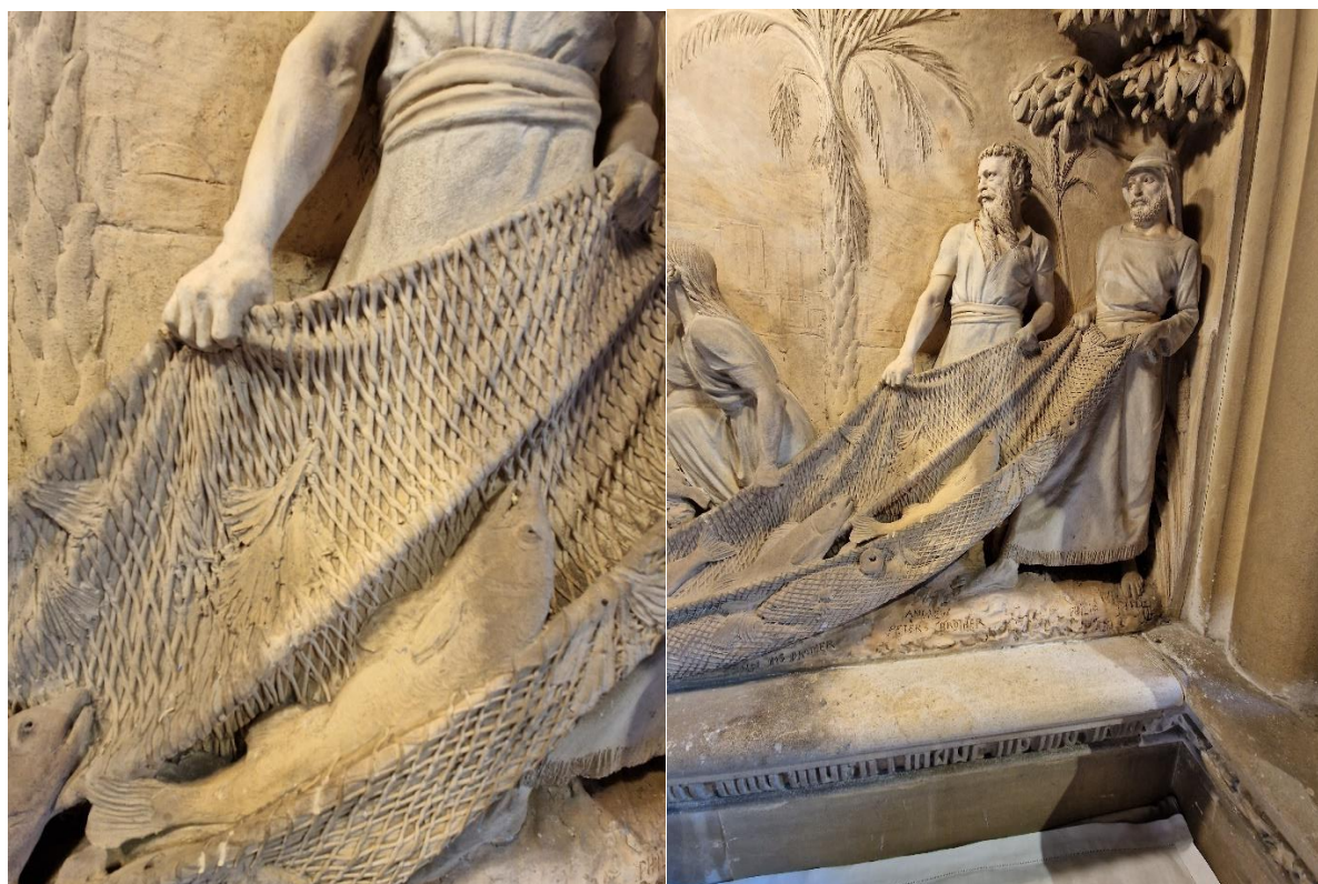
Figures 22 and 23. Cleaning trial to complex surfaces of terracotta.
