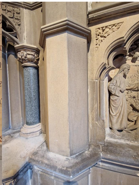
Figure 25. Stone pier and spandrel to panel cleaned.
