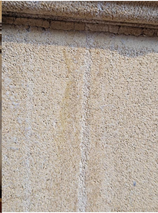
Figure 3. Condensation run-off pitted corrosion.
