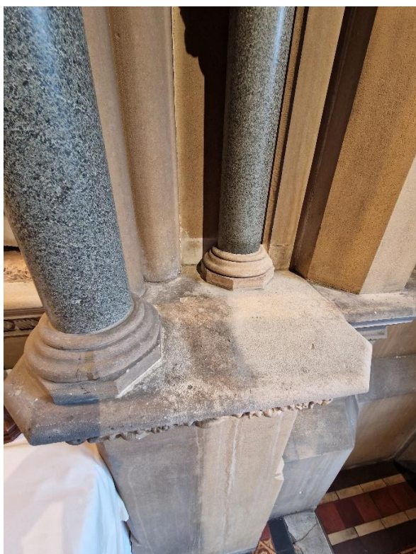
Figure 28. Part cleaned shaft base and shelving.
